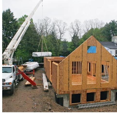
**A crane provides muscle.** Most of the time, walls can be tilted up by hand. However, for staging and stacking panels, tilting up large gable-end walls, and placing roof panels, a crane or a large forklift is a must.
