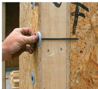
Electrocoated SIP screws with broad tin washers fasten the corner joints where dimensional lumber is installed. Midwall joints use splines that are slipped into channels routed in the foam. Splines are secured with 6d ring-shank nails; then expanding foam is inserted into the center channel to seal the joint.
