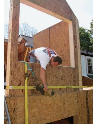
**Panels are moved into place with lifting plates and straps.** Steel lifting plates are screwed to the skin of wall and roof panels. Nylon webbing attaches to the pin on each plate. A crane or forklift grabs the webbing to move the panel where it needs to go. Manually operated ratchet straps have literally tons of pulling strength. Straps are essential for finessing large panels into difficult spots and for holding them in place while fastened.
