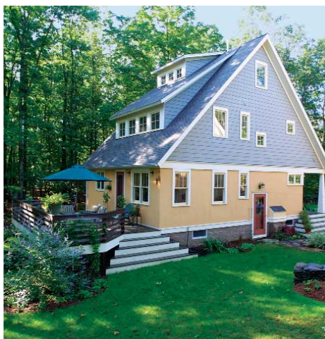
A modern American house with European origins. A combination of Swiss stacked dormers, deep overhangs and a Craftsman sensibility, this design combines good use of space with inexpensive materials. Photo facing page taken at A on floor plan; photo above taken at B on floor plan.
