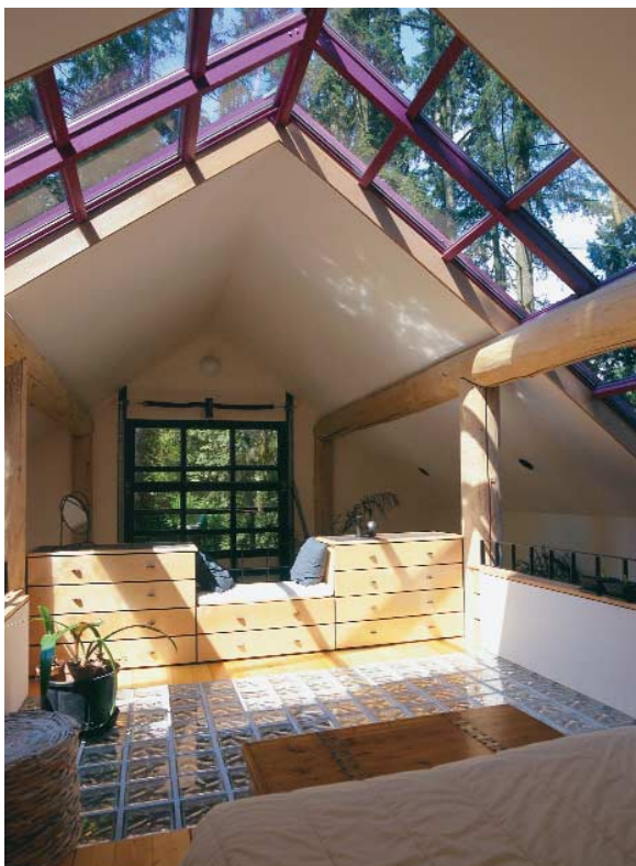
A glass-block floor lets the light through. Mounted in a custom-fabricated 675-lb. steel grid, the glass blocks allow sunlight from the skylight above to pass through the floor of the sleeping loft and onto the living area below. Photo taken at C on floor plan.
