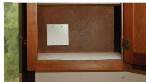
**SOLUTION** Find a spot where the splice box is accessible and still not obvious. In kitchens, try mounting a box slightly above the upper cabinets. Unless the room is enormous, you will never see it. If the cabinets go to the ceiling, mount a box in the back of the cabinet; the only part you will see is a flat blank plate.
