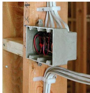
**SOLUTION** Wiring passing through holes closer than 1¼ in. to the framing face must be protected with nail plates. Several runs of wiring can be corralled with inexpensive Cable Stackers, which maintain the distance mandated by code.
