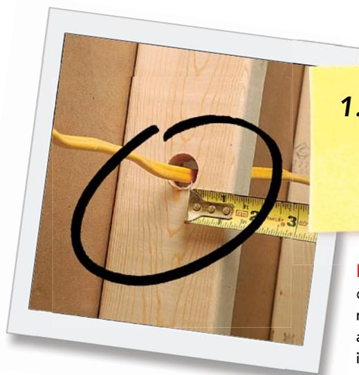
**1. Protect wiring from nails and screws.**
