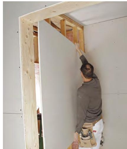
**Hang it short.** When a single panel will cover a wall or ceiling end to end between walls, cut it about  $\frac{1}{4}$  in. short so that it goes between the walls easily without binding on the framing.
