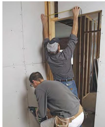
**Fill in with cutoffs.** Don't cut full panels to fill small gaps. Leave the spaces empty, and come back later to fill in with scraps from larger pieces.
