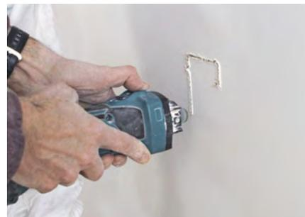
**Mark for boxes.** Electrical boxes are typically all at the same height. Measure a few to be sure, then mark the location of each on the floor directly below. When the panels go in, just measure up and quickly make the cutouts.
