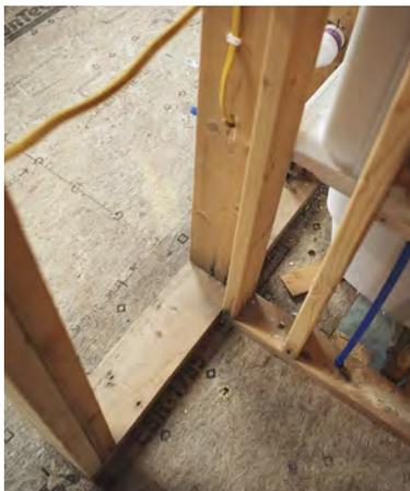
**Nailer needed.** You can safely float corners up to 8 in., but a short wall section like this requires a nailer.
