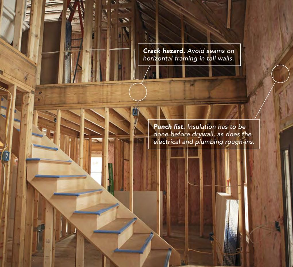
**Crack hazard.** Avoid seams on horizontal framing in tall walls.
