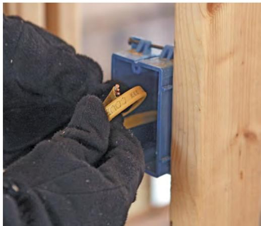
**Safety first.** Electrical cables need to be pushed into the back of boxes before the drywall is hung to avoid getting nicked by cutting tools.
