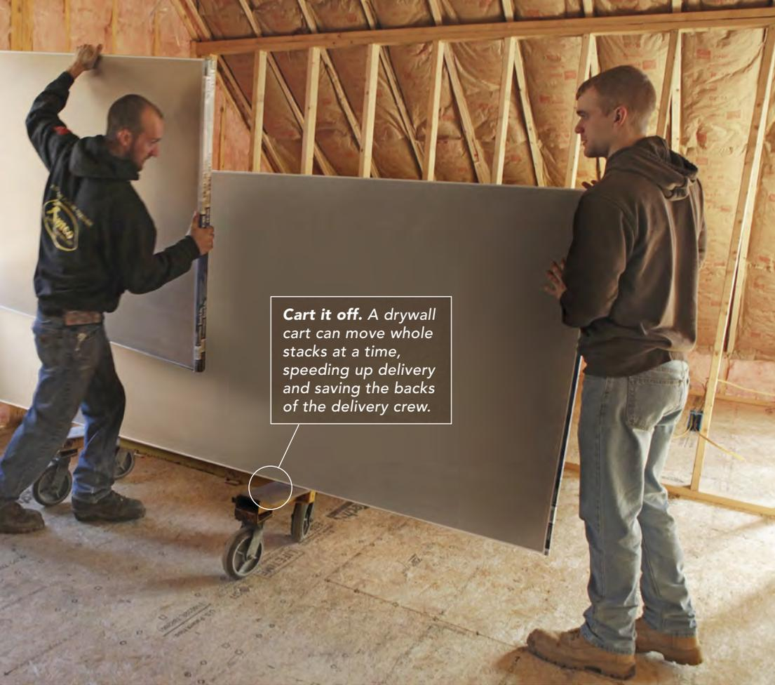
**Cart it off.** A drywall cart can move whole stacks at a time, speeding up delivery and saving the backs of the delivery crew.
