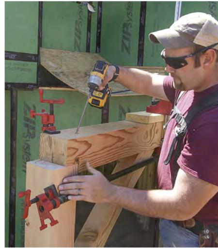
**Fit the braces.** After coercing the braces into their mortises, pull everything tightly together with a pair of clamps, and then secure the post-to-beam connection with long structural screws driven at an angle.
