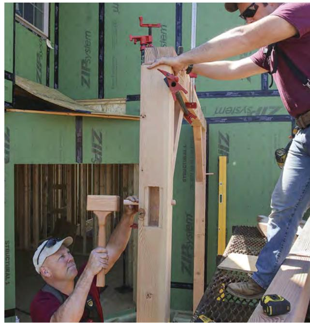
**Hammer it home.** Working as a team, have one person brace the frame while the other pounds the 10-in.-long, rounded-tip oak peg into place with a mallet. Later, the pegs can be trimmed to length, either flush or slightly proud.
