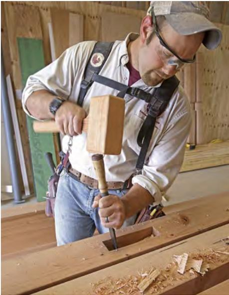
**Chisel it square.** Use a large, heavy chisel and some enthusiastic swings of a mallet to remove the remaining waste wood and square up the four sides of the mortise, making sure the bottom is relatively flat.
