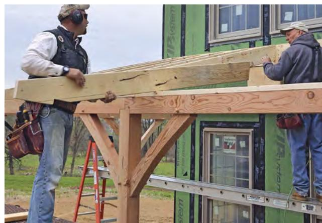
**A stick-framed roof.** Although a timber-framed roof is a common way to top this style of porch, it's not the only way to go. If the roof framing will be concealed, it's easiest to finish up with conventional 2x framing lumber.
