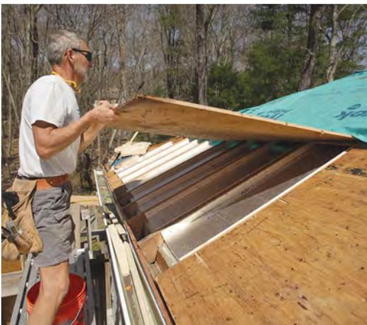
**Drop the hood.** After the insulation, baffle, and sealing work is done, drop the sheathing back down and nail it off. Avoid old nail holes for solid fastening.
