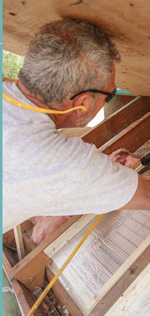
the baffles up the slope. The wood strips, meanwhile, act as spacers to keep the top of the baffles  $1\frac{5}{8}$  in. or more beneath the roof sheathing, and also as a means to attach the baffles to the rafters.
