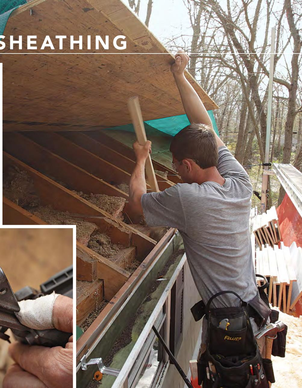
**Punch them through.** Specialty nail-removal tools are available, but you can also make your own by grinding the nose of an old framing nailer, allowing it to punch the sheathing nails through the sheathing to release each sheet from the rafters. We ground  $\frac{3}{8}$  in. of metal from the nailer's nose, and the driver (which strikes the nail) now projects  $\frac{5}{8}$  in.
