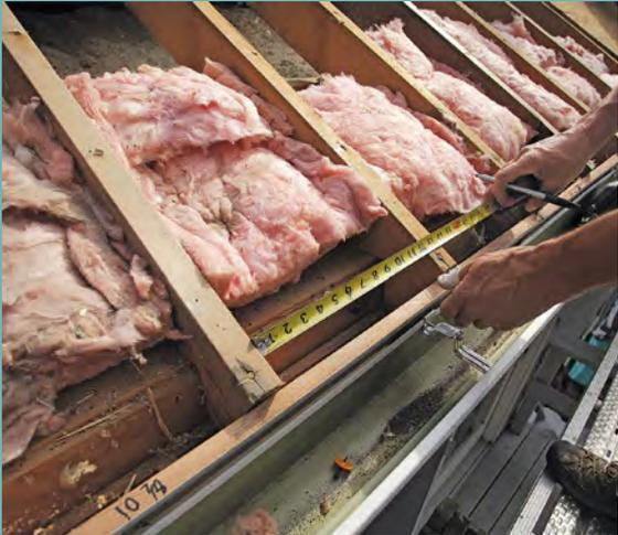
**Foam and furring strips.** Measure each rafter bay at the bottom and 4 ft. up, take the lesser of the two measurements—as long as they're less than  $\frac{1}{4}$  in. different—and write it on the fascia or top plate. If the measurements vary by more than  $\frac{1}{4}$  in., you'll need a tapered baffle. On the ground, cut the 1-in. foam using a track saw, and attach wood strips on either side using  $\frac{1}{2}$ -in.-crown by  $1\frac{3}{4}$ -in.-leg staples.
