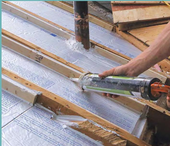
**Notch for joists.** Where ceiling joists get in the way, cut the foam to fit around them, and use shorter wood strips in some cases. Fill any gaps with caulk to aid in preventing wind-washing of the insulation below.
