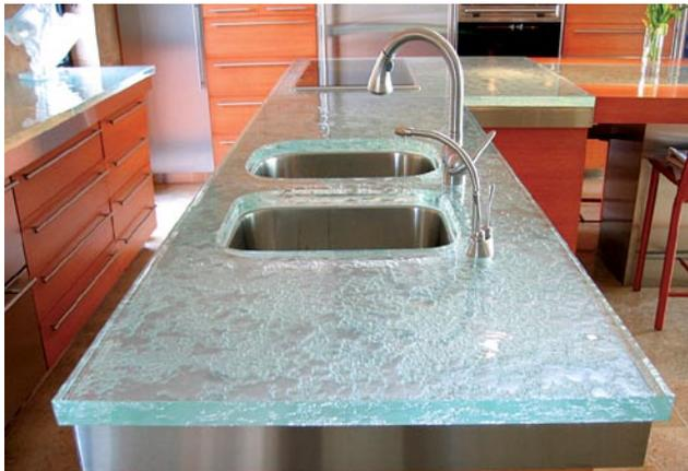
more than 2 in. thick. Kiln-fired tops can be made only as large as the kiln that fabricators have access to, typically 6 ft. wide by 12 ft. long.
