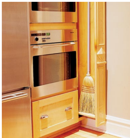
STORAGE DETAILS , like this pull-out column for brooms, make efficient use of extra space. Similar columns to house spices and baking ingredients and even containers for trash and recyclables were built in elsewhere.
