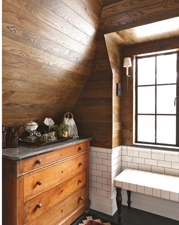
Finish work. The angled ceiling of the master bath is finished with white-oak planks that put craftsmanship on display.
