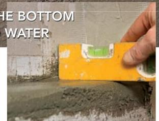
Trowel a ½-in. layer of mortar in the bottom of the niche, and use a level to make sure it has a slight pitch. Slant the bottom of the niche just enough so that water flows out of it, but not so much that bars of soap and bottles of shampoo slide out. I aim for a ⅛-in. slope over 3 in.
