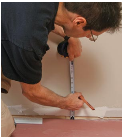
The bottom rail is wider than the top rail. The distance from the top of the bottom rail to the top of the baseboard, which will be added later, should be equal in width to the top rail. In this case, the top rail is 2½ in. wide, and the baseboard will be 3½ in. wide. I snap a line 6 in. off the floor and cut a piece of drywall 6 in. wide to get the proper proportions.
