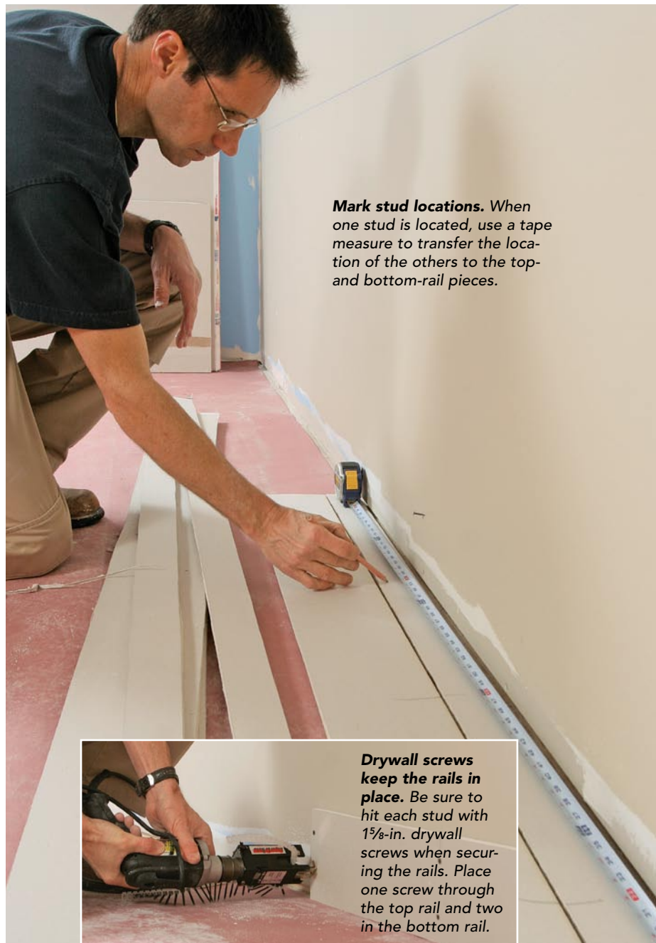
Measure, mark, and snap a level line around the room. Hold the wainscot's top rail to this line to be sure all the panels are level.
