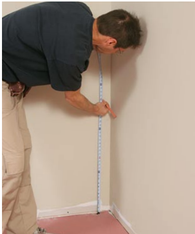
Measure, mark, and snap a level line around the room. Hold the wainscot's top rail to this line to be sure all the panels are level.
