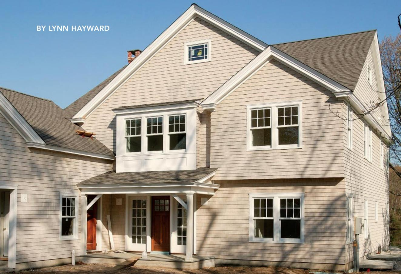
**S**idewall shingles and clapboards have nuances and limitations, but they share the same goals. Besides shedding water and protecting a structure, siding enhances the architectural lines of a house. Each course should run level around the building, align at inside and outside corners, and end where it began.
