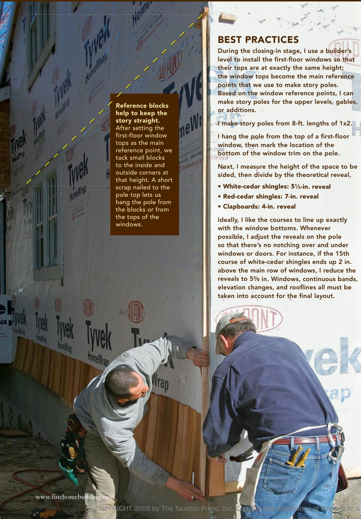
**Reference blocks help to keep the story straight.** After setting the first-floor window tops as the main reference point, we tack small blocks to the inside and outside corners at that height. A short scrap nailed to the pole top lets us hang the pole from the blocks or from the tops of the windows.
