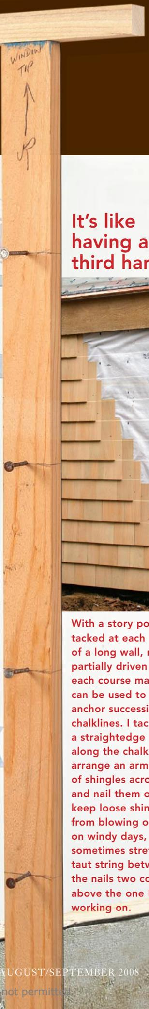
With a story pole tacked at each end of a long wall, nails partially driven into each course mark can be used to anchor successive chalklines. I tack a straightedge along the chalkline, arrange an armful of shingles across it, and nail them off. To keep loose shingles from blowing off on windy days, I sometimes stretch a taut string between the nails two courses above the one I'm working on.
