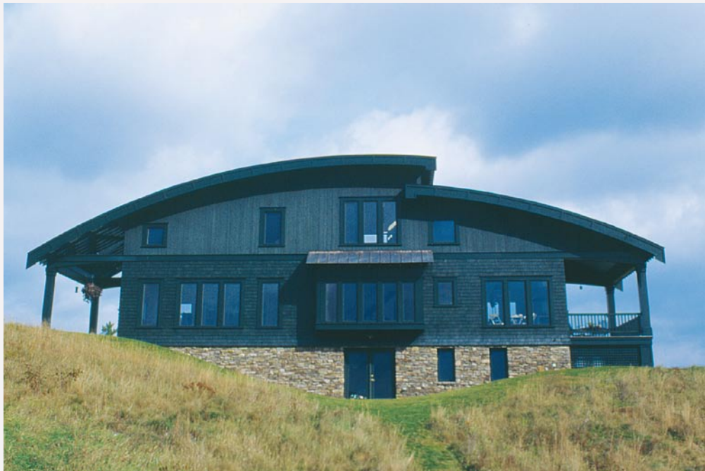
Arc of the roofline is broken to admit light. When the authors realized that their first roof design of a single parabola would create a somewhat dark middle bedroom upstairs, they stepped down one portion and added clerestory windows in the intervening space. Photo taken at C on floor plan.
