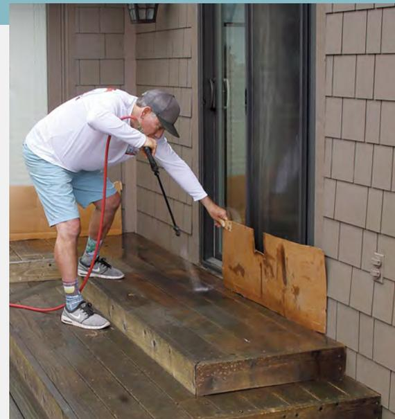
**Protect metal.** The cleaner and oxalic acid can etch metal, including aluminum-clad windows and doors, so protect them with plastic sheeting or cardboard. The cleaner can also leave water spots on glass if allowed to dry, so rinse any overspray off of windows and doors as soon as possible.
