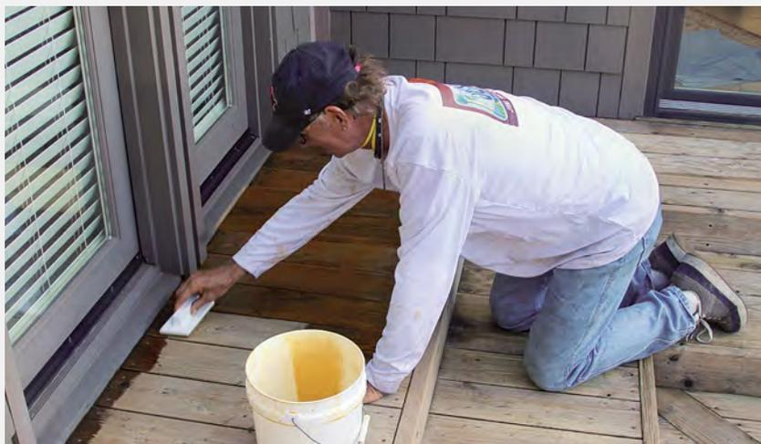
**Cut in.** Use a brush or painting pad to cut in along the house and anywhere else at risk of overspray from the airless sprayer used for the rest of the deck. I prefer a pad because it holds more finish than a brush.
