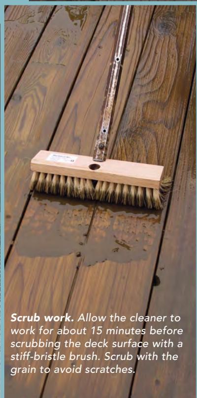
**Scrub work.** Allow the cleaner to work for about 15 minutes before scrubbing the deck surface with a stiff-bristle brush. Scrub with the grain to avoid scratches.
