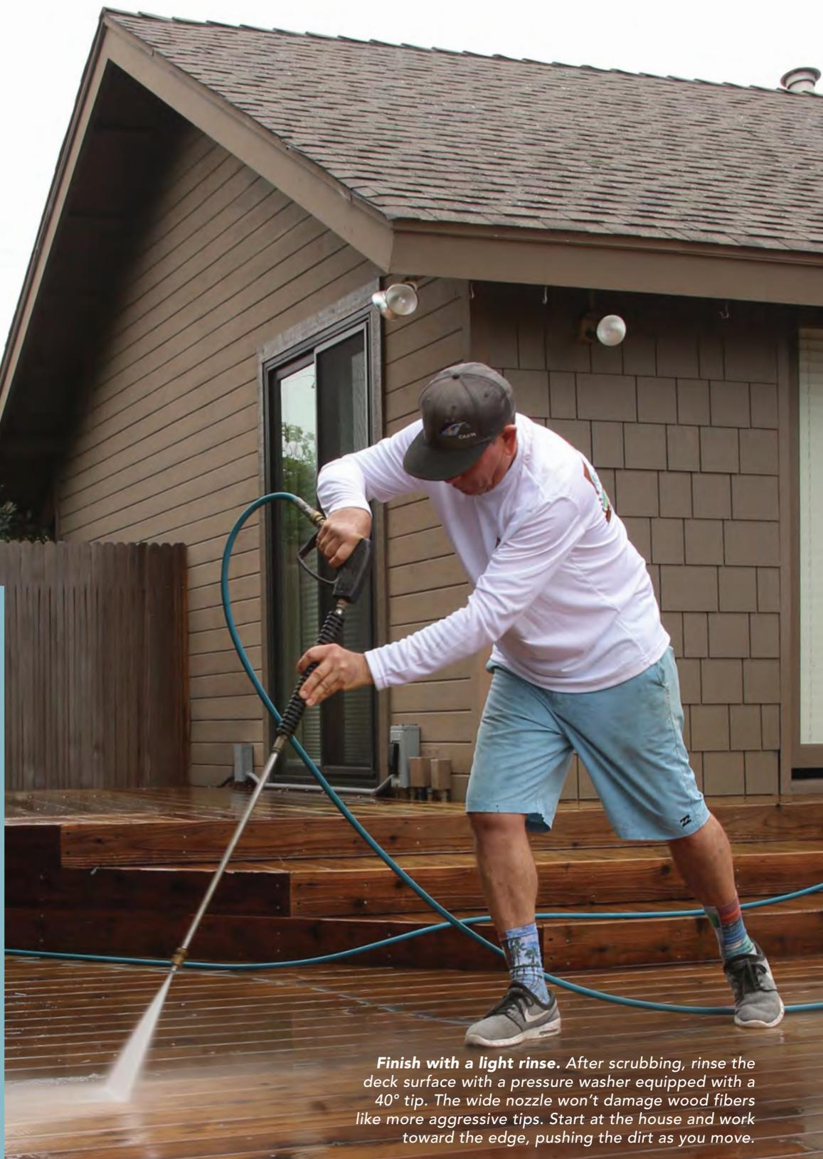
**Finish with a light rinse.** After scrubbing, rinse the deck surface with a pressure washer equipped with a 40° tip. The wide nozzle won't damage wood fibers like more aggressive tips. Start at the house and work toward the edge, pushing the dirt as you move.
