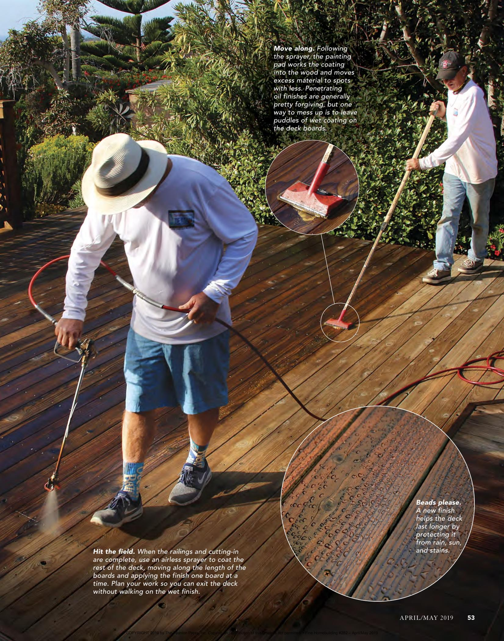
**Move along.** Following the sprayer, the painting pad works the coating into the wood and moves excess material to spots with less. Penetrating oil finishes are generally pretty forgiving, but one way to mess up is to leave puddles of wet coating on the deck boards.
