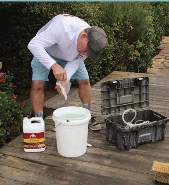
**Mix a batch of cleaner.** One gallon of wood-brightening cleaner and 4 gal. of water make 5 gal. of cleaner, which is enough to clean about 400 sq. ft. of decking. Adding 1 oz. of oxalic acid crystals per gal. of water makes the solution better at brightening weather-beaten wood.
