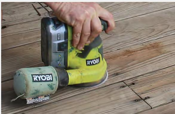
**Sand rough spots.** Sanding the whole deck is unnecessary, but split or checked boards should be sanded to prevent painful splinters. Ensure fasteners are driven below the deck surface before sanding.
