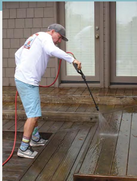
**Apply the cleaner, let it work.** Although a garden sprayer works, it can be tedious to constantly pump. Instead, I apply the cleaner with an electric-powered agricultural sprayer so it fully coats the deck surface and railings. For more on this setup, visit [FineHomebuilding.com/magazine](http://FineHomebuilding.com/magazine).
