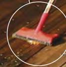
**Hit the field.** When the railings and cutting-in are complete, use an airless sprayer to coat the rest of the deck, moving along the length of the boards and applying the finish one board at a time. Plan your work so you can exit the deck without walking on the wet finish.
