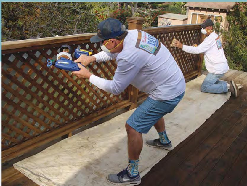
**Start at the top.** Vertical surfaces and anything above the deck get coated before moving to the deck surface. A small airless sprayer is great for coating railings, but once the coating is sprayed, work it into the surface and absorb any excess with a painting pad.
