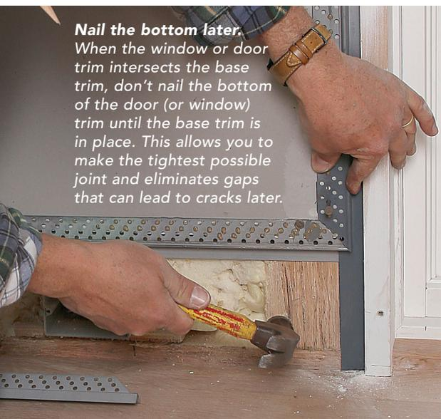
**Nail the bottom later.** When the window or door trim intersects the base trim, don't nail the bottom of the door (or window) trim until the base trim is in place. This allows you to make the tightest possible joint and eliminates gaps that can lead to cracks later.
