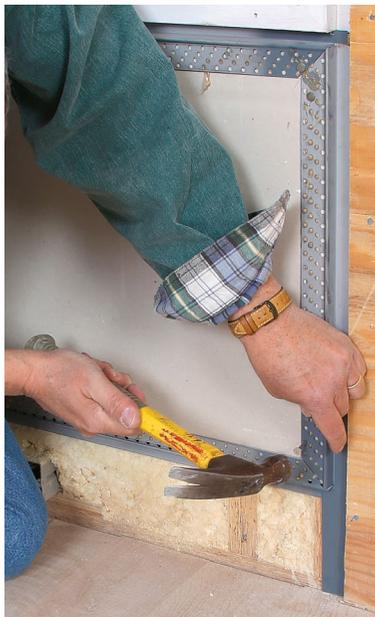
**Nail it up.** In addition to construction adhesive, the reglet trim is held with ring-shank nails made for exterior stucco trims like weep screed and outside corners. They have a thicker shank and deeper rings than drywall nails.
