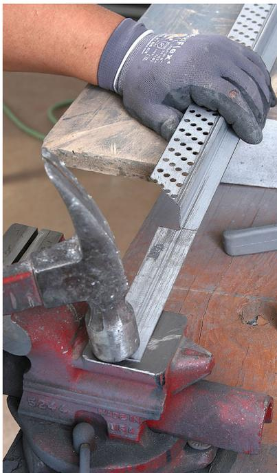
**Metalwork.** A small bench vice, a smooth-faced hammer, and hand benders help with fabrication. This piece of reglet intersects with a piece of base trim; we flatten the “L” so the poplar base can overlap without gaps.
