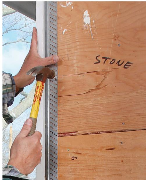
**Making transitions.** Although reglet offers no structural support, it often acts as an important visual transition between different materials. On this house it replaces casing, acts as the transition from wall to baseboard, and transitions between stone veneer columns and the walls.
