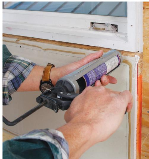
**Use glue too.** High-quality solvent-based construction adhesive holds the reglet trim better than nails alone. This helps prevent the movement that can cause cracks in the joint compound applied on top of the trim. The pencil lines from the dry fit show where to put the adhesive.
