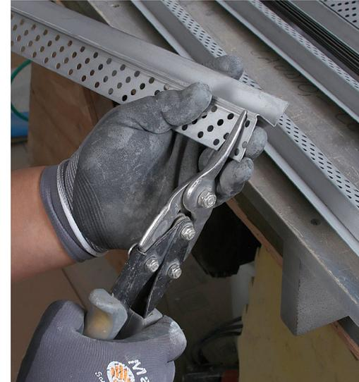
**Use snips for small cuts.** High-quality aviation snips also work for cuts. Wear gloves when handling the pieces because even the factory-cut edges are razor sharp.
