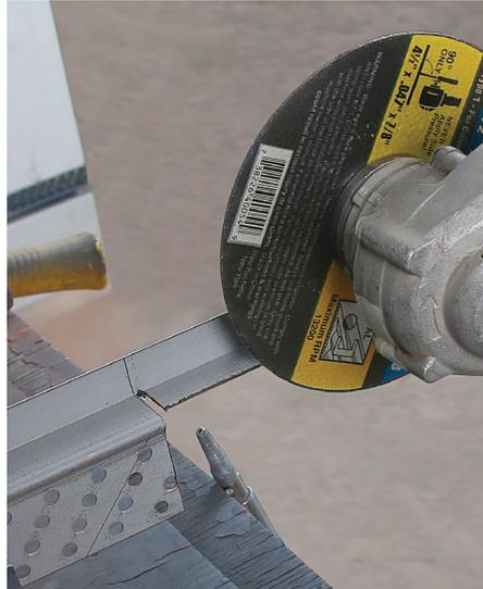
**Use a grinder for rip cuts.** An angle grinder with a steel-cutting abrasive blade is best for removing flanges and making stopped cuts. Remove burrs with a file or wire brush so joints are tight.
