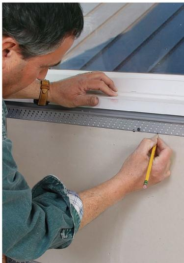
**Dry-fit first.** After cutting, dry-fit the reglet parts using drywall screws to temporarily hold them in place. Adjust the fit until all the miters are tight and then mark the inside perimeter to guide the placement of construction adhesive.
