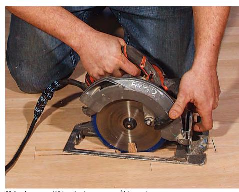
**Make three cuts.** With a circular saw set to  $\frac{3}{4}$  in., make two cuts down the length of the board and one at an angle across (an "N" shape). This releases pressure and makes removing the pieces easier. Be sure to make the first cut to the inside of any nails, then move over an inch and make the second lengthwise cut.
