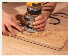
**Go slow.** Use a router to remove the top one-third of the board surface in <sup>1</sup>/<sub>16</sub>-in. increments. Rout down to just above where the tongue and nails sit.
