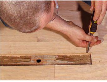
**Pry the tongue.** Remove the tongue of the cut board from the groove on the adjacent board.
