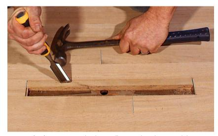
**Remove the damage.** Use a chisel or oscillating multitool to extend the lengthwise cuts to the ends to free the center strips, and remove them; the groove side should come out easily. Use a hammer and chisel to chip away the tongue side, and use a cat's paw to remove any nails.
