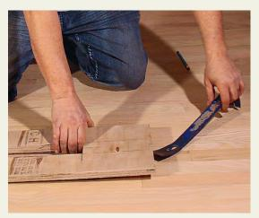
Check the match. Remove the template, clean up the corners with a chisel, and do a dry fit, gently tapping the replacement piece into place to ensure it is reasonably flush. For final installation, lay in the adhesive, tap the board into place with a rubber mallet, weight it until the glue sets, and then sand if needed.
