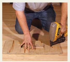
**Set a guide.** Nail a <sup>3</sup>/4-in. plywood template over the area so the router bit and bearing ride on the template without hitting adjacent boards. If the floor is already finished, either tack the template between board seams or use double-sided tape to hold it down. Do a test to make sure the tape won't mar the floor.
