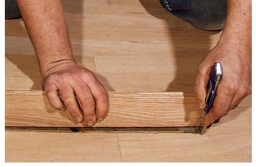
Mark, cut, check. Use a utility knife to mark the cut on the replacement board. Cut it to size and dry-fit, laying dental floss or a piece of paper down first to make it easy to remove.
