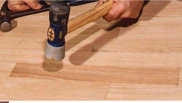
**Tamp it in.** With a rubber mallet, gently tamp the new board in place. Weight the new board until the adhesive sets up.
