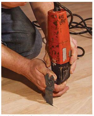
Mark the repair. If it's a long board, mark the section being replaced with a square. Use an oscillating multitool to make the first two cuts at both ends of the damaged area.
