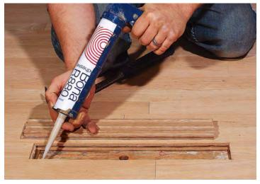
**Anchor the board.** Apply adhesive (we use Bona, but Liquid Nails or yellow glue work too) to the tongue and groove of the adjacent boards, and slide the replacement piece into place. Do not glue directly to the subfloor.
