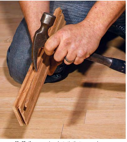
**Modify the groove.** In order to tip the tongue-and-groove replacement board into place—tongue-side first—rip the back of the groove with the claw of a hammer to make a rabbeted joint.
