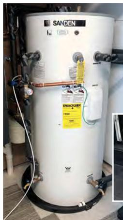
**Most heat-pump water heaters combine the heat-pump compressor and tank in an integral unit. Sanden's SanCO<sub>2</sub> is unique in the U.S.—it's a split system with the storage tank inside the house and a separate compressor outside. Even more unique is the fact that it uses CO<sub>2</sub> as the refrigerant rather than a hydrofluorocarbon.**
