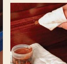
**Last-minute touch-up.** I like to fill imperfections and nail holes after the first topcoat so that the putty matches the wood tone exactly. Force the material into the hole; then wipe it clean. You might need to mix two or three colors to match various tones in the piece.
