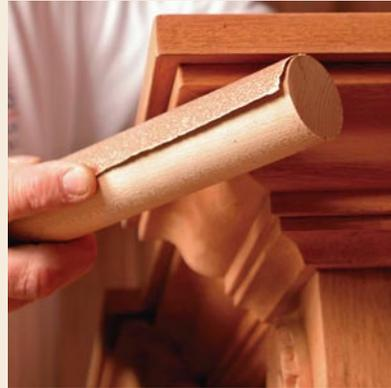
**Ease sharp edges, but don't alter the profile.** Sharp joints and edges splinter easily and don't take finish well. Use gentle pressure, and sand in the direction of the grain. Sandpaper wrapped around a wooden dowel works well on crown, especially in the cove portion of the profile.
