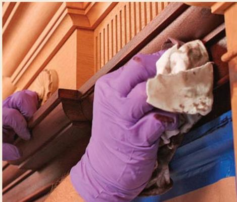
**Wipe with a clean rag.** As you're working across the surface, keep the soaking time consistent for all sections, and pay attention to the edges, profiles, and corners. Replace the cloth when it gets loaded with stain.
