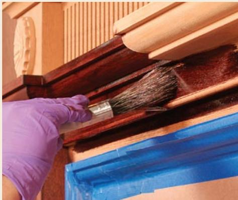
**Cut in with a brush.** Working in small sections, apply the stain liberally, and let it sit for several minutes before wiping it off. Apply stain in a neat, orderly process. Excess stain can drip, run, and puddle, which can leak or leach out from behind moldings afterward.
