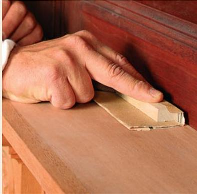
**Hit the imperfections first.** The area around an errant nail becomes a lump in the surface. To flatten it, use 120-grit sandpaper wrapped around a flat, square-edged block. Once all imperfections are sanded, begin sanding the entire surface.
