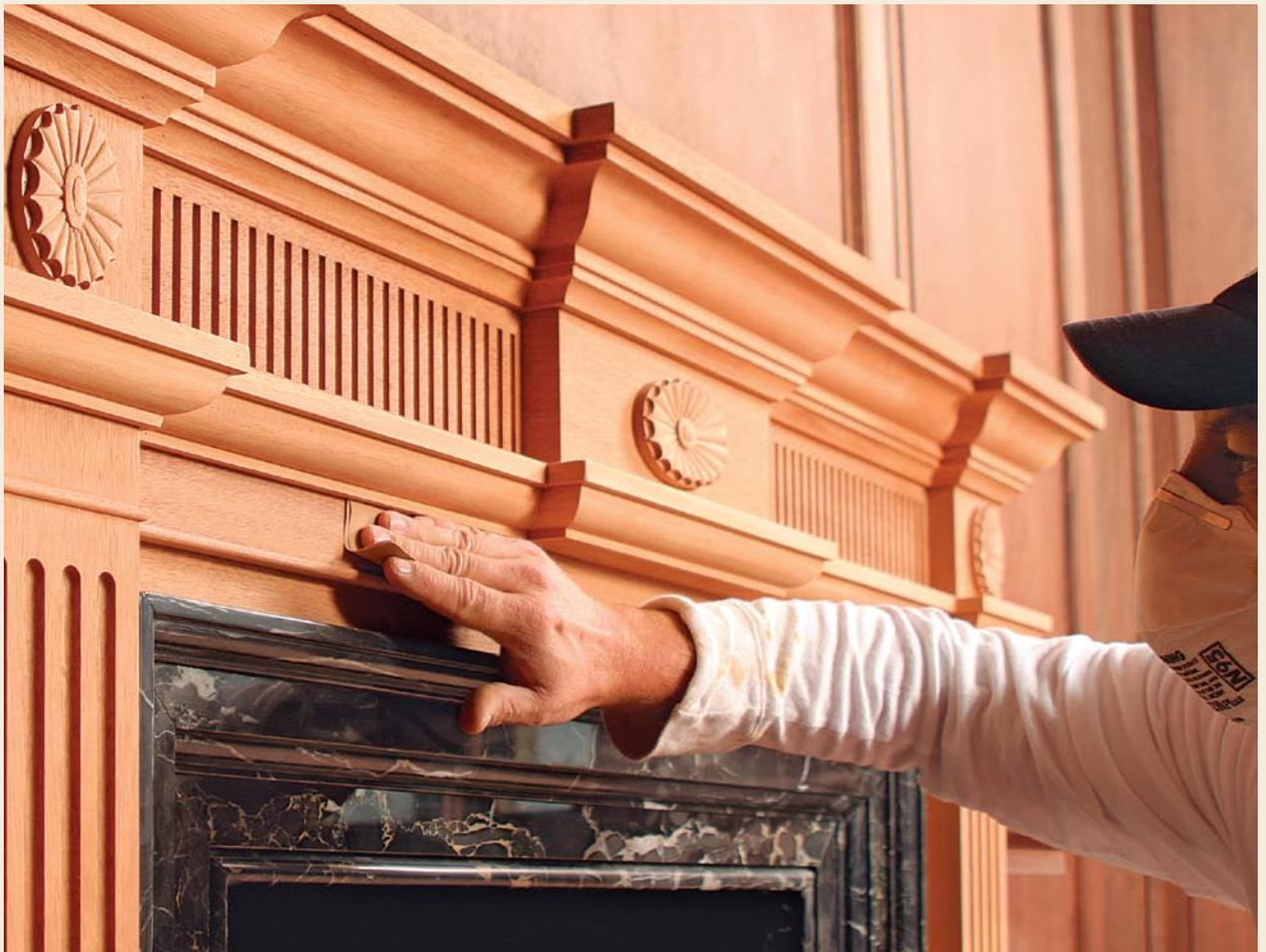
**One section at a time.** Sand each shape or plane separately so that you don't sand one spot more than another or in the wrong direction relative to the grain. Be sure to get into grooves and crevices, and around corners. Keep the area well-lit and vacuumed so that you can see the surface. Make sure everything feels smooth before proceeding to Step 2.
