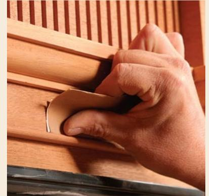
**Sand every inch, no matter how smooth it looks.** Planer and profile-cutting knives compress the top layer of wood fibers so much that stain can't penetrate the surface the way that it's designed to. That's why it's necessary to sand everything before applying stain.
