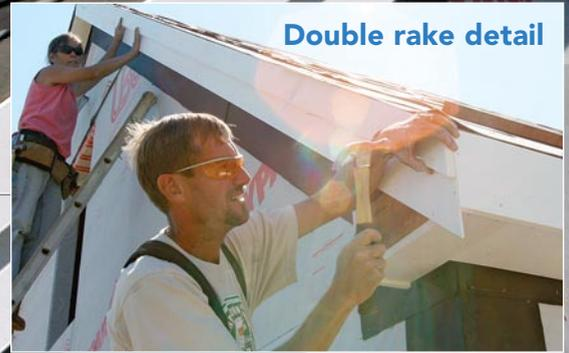
To hide any irregularities in the rake boards, such as gaps caused by rafter crown, I install a double member. I measure up from the bottom edge of the rake boards and snap a chalkline to guide the installation. If I know there will never be a gutter, I use a beveled double member on the fascias as well. If you use this detail, remember to allow visually for the coverage of the drip edge when sizing it.
