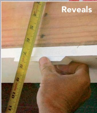
To help keep the reveal on the fascias and returns consistent, I rip a 3/8-in. gauge block that I keep in my tool belt throughout the installation. I use it as a reference when measuring the height of the rake boards and again as a guide when assembling the fascias and returns.
