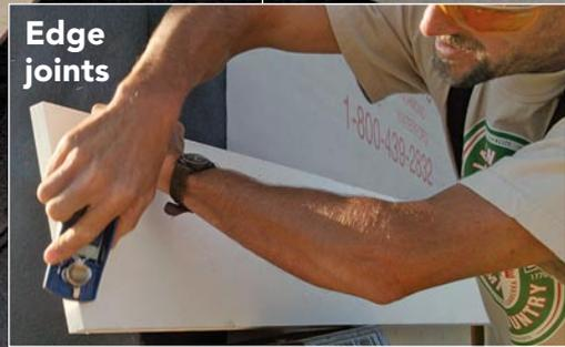
The only time I use butt joints on exterior trim is when piecing together eave soffits. PVC doesn't get putty and paint, so I chamfer the edges with a block plane to soften any potential shadowlines from a joint that isn't perfectly matched. To help shed water, fascias are pieced together with scarf joints (drawing right), and the rakes are oriented so that the upper piece laps over the lower one. Leave the outer bevel just a whisker long; then force the joint in place.
