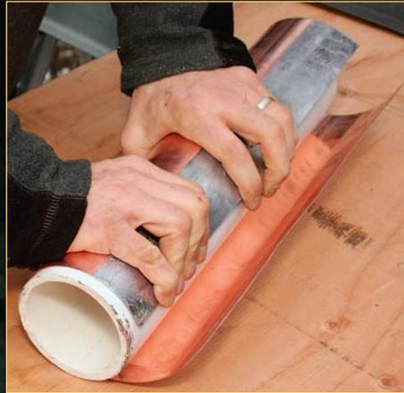
**Spin it.** Wrap the sleeve stock around a scrap of PVC that's the same size as the vent pipe. Roll it gradually and slowly to avoid kinking the copper.
