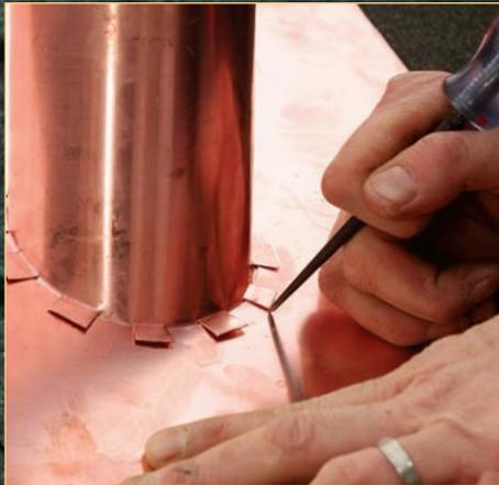
**Test-fit the boot.** Lock the sleeve to the pan with the 1/2-in. tabs, then slide the boot over the vent pipe. Square the pan to the shingles. Then rotate the sleeve until it sits correctly. Finally, scribe the tabs to mark their exact location.
