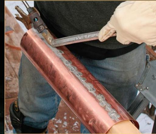
**Solder the joint.** Tack the joint every 2 in. first to hold it together. Then run a thick bead of solder down the length of the joint.
