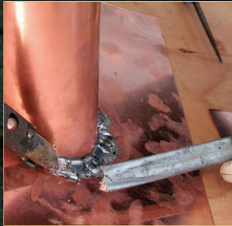
**Run a heavy bead.** After tacking the tabs to the pan, seal the joint with a heavy bead of solder. Work slowly, taking care not to overheat the metal. If solder starts to run through the joint and beneath the pan, take a break until the piece cools.
