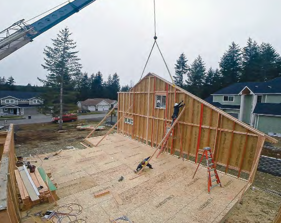
Made for lifting. Rather than put the wear and tear of lifting walls on our own bodies, we put it on machines made for the job.
