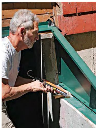
**POSITION, SHIM, AND SEAL** Shim the whole unit about 1 in. above the foundation and apply a bead of sealant along the foundation and walls for the new door frame to bed into.
