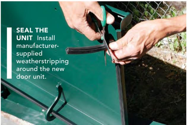
**SEAL THE UNIT** Install manufacturer-supplied weatherstripping around the new door unit.
