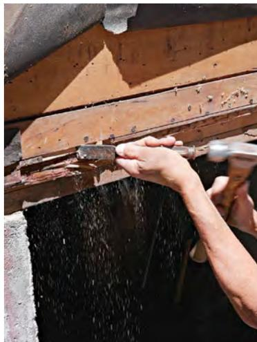
**TRIM THE SHEATHING** Use a circular saw with the blade set at the depth to be removed to cut along the flange mark, and follow up with a chisel to remove the remaining material to recess the flange.
