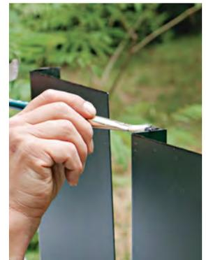
**CUT TO FIT** I cut the plates with a tungsten carbide metal-cutting blade in a circular saw; an angle grinder with a cutoff wheel can also be used. Prime and paint all cut edges.
