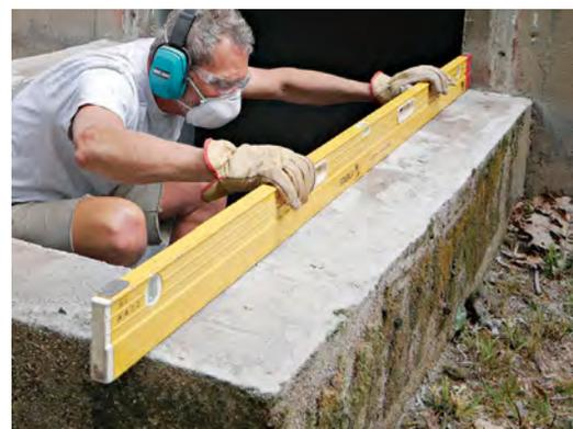
**CHECK FOR LEVEL** Before installing the new door, use a long level to check the foundation for level in all directions. If needed, apply a concrete resurfacer to level out low areas, or use a grinder to level out high spots.
