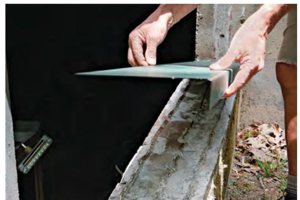
**INSTALL THE PLATES** Apply a thick bead of high-quality sealant to the top of the clean foundation before installing the plates.
