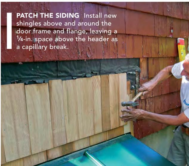
**PATCH THE SIDING** Install new shingles above and around the door frame and flange, leaving a 1/4-in. space above the header as a capillary break.
