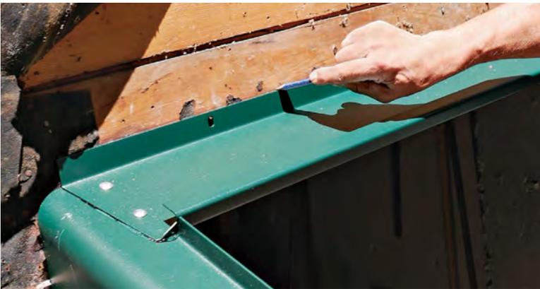
**DRY-FIT THE FRAME** Center the frame on the foundation and check the seal against the house. Here the  $\frac{3}{4}$ -in. sheathing was about  $\frac{3}{8}$  in. proud of the concrete, so I traced the flange on the wall for a cutline.
