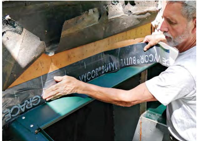
**MANAGE WATER** Apply self-adhered flashing tape over the header flange of the door, tucking it beneath the water-resistant barrier on the wall.
