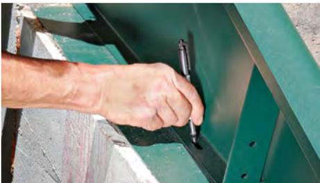
**PREPARE FOR DRILLING** Locate and mark the mounting holes on the foundation and walls.
