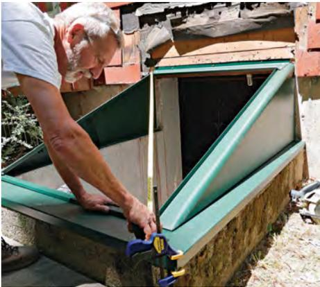
**PLUMB AND SQUARE** Dry-fit the door tight against the house and centered on the foundation plates. Measure diagonals to verify that the unit is square, adjusting as necessary.
