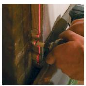
**SINK ADDITIONAL SCREWS** Without moving the laser, drive another screw near both the top and bottom of that same stud, stopping when the mark on the bit holder aligns with the laser.
