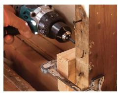
**BLOCKS LOCK IT IN** After repeating the process on the other end of the wall, set blocks alongside the studs at each screw position. Set the face of the blocks in plane with the screwheads, and use a clamp to ensure they don't drift off the mark while being fastened.
