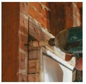
**ORIENT THE LASER** With the bit back in the holder, position the drill as if you were driving the screw while a helper sets up a plumb laser line at the other end of the wall. Adjust the laser line until it aligns with the mark.
