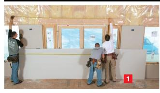
Along with all the standard headers and blocking, a wall this big will probably have a framing transition halfway up, too. All these things lead to bumps and dips in the wall—bad places to put seams or lots of fasteners.
