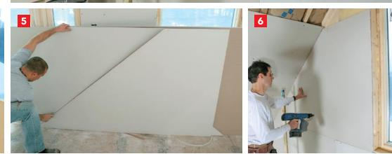
had been less than 48 in., I could still rip a sheet to fit the width. If it were more than 48 in., a 54-in.-wide sheet of drywall could be ripped as necessary. Any wider than 54 in., though, and a horizontal seam is a must.
