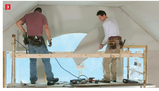
are most likely to move over time, and movement will lead to screw pops. I keep screws about 6 in. down from where the wall meets the ceiling for the same reason.
