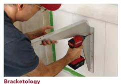
Aluminum brackets from A&M Hardware are screwed to wall studs. Weighing only 4 lb. each, the two brackets support over 1400 lb. together under load testing.
