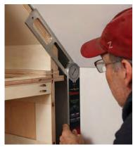
Scribe the face-frame parts The face frame is scribed to the ceiling with an angle finder. The angle is transferred to the miter saw for a matching cut.
