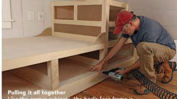
Like the corner cabinets, the bed's face frame is installed as a unit, pocket-screwed from behind, except for the bottom, which had to be face-nailed.
