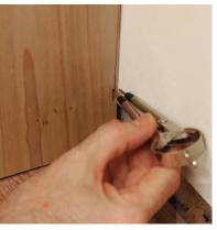
Scribe, scribe again Scribed to the wall with a compass and to the floor with a scrap of new flooring, the side and bottom edges are trimmed with a jigsaw.
