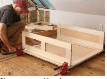
Clamps as a workbench The bottom web frame is glued up with parallel bar clamps, which proved to be a solid, stable platform for the rest of the cabinet build.
