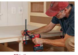
Fill in the gap With the plywood bed planks installed, cleats are installed between drawer dividers to add rigidity behind the face frame at the front edge of the bed.
