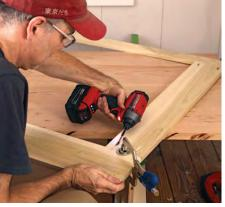
Assemble the face frame The parts scribed to the wall and the floor are pocketscrewed together. The assembly is then clamped in place while subsequent parts are cut and fit one at a time. The last piece of the puzzle is a triangular <sup>1</sup>/<sub>4</sub>-in. MDF panel set into grooves cut in the same fashion as the webframe joinery.
