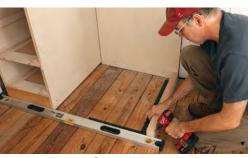
**Square the opening** A plywood mounting block is squared flush with the front of the corner cabinet and pocket-screwed to the floor.
