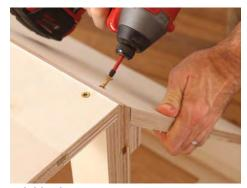
Solid backup The angled subtop is screwed from the outside with angled cleats holding it in position. It and the short outer support are the only solid <sup>3</sup>/4-in. plywood components.
