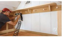
A touch of Shaker trim A 10-in.-deep shelf is pocket-screwed from behind to the peg board before the assembly is nailed to wall studs.
