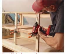
Top off the framework The subtop is fastened in the same way, while drawer runners for the upper drawers are glued and clamped in place.
