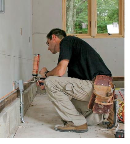
"Spray foam is a fantastic air barrier where it is," Ueno says. "It does nothing where it's not. So any time you have a wood-to-wood joint where it's not covered up by the spray foam, all of those are potential air-leakage locations."
