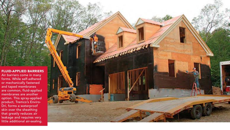
be strong, durable, continuous around the entire building enclosure, and, of course, air impermeable. "Air barriers keep outside and inside air out of the building enclosure," Joseph Lstiburek wrote in a paper published by the Building Science Corporation. "Air barriers can be located anywhere in the building enclosure—at the exterior surface, the interior surface, or at any location in between."
