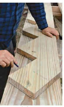
**Use the first stringer as a template.** Align the straight edge of the template to the new stock, and hold it firmly in position. Use a sharp pencil to transfer the layout.
