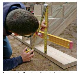
Incorporate the slope. Extend a level across the first step of the first stringer. Measure the distance to the plate at the location of each additional stringer, add the plate thickness, and cut the heel before notching for the heel plate.
