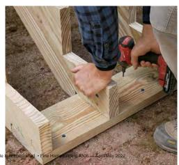
Lock down the heel plate. Use a mason's bit to drill holes through the plate and into the brick. Then drive concrete screws, two between each stringer, to lock the plate into position.
