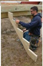
Notch the heel to fit the **plate.** Use a circular saw followed by a jigsaw to cut an accurate notch for receiving the 2x10 plate that will tie the assembly together. Dry fit both pieces, and check that the treads are still level.
