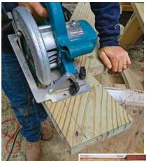
Cut the heel and check the fit. The first heel cut matches the thickness of the decking. Make the cut, then position the stringer so that it's tight against the carrier beam and snug to the band joist above. Use a torpedo level to ensure treads are level.
