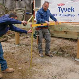
Find the overall rise. At a central location across the deck frame, we used a level to extend the deck height outward 55 in. At this point we found the grade 3 in. lower than at the edge of the 42-in-high deck frame, for an overall rise of 45 in.
