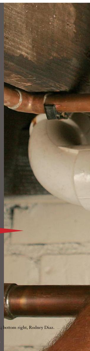
over time, especially in tees, 45° elbows, and 90° elbows, which are subject to significant force as water flows. Water slowly eats and erodes copper in these areas. Improper soldering techniques are also a common source of leaks.
