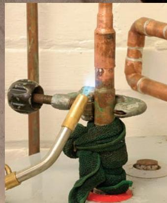
soldered, I try to solder the farthest ones first to avoid scalding myself. I also make sure to open all shutoffs that will be heated to avoid damaging washers.
