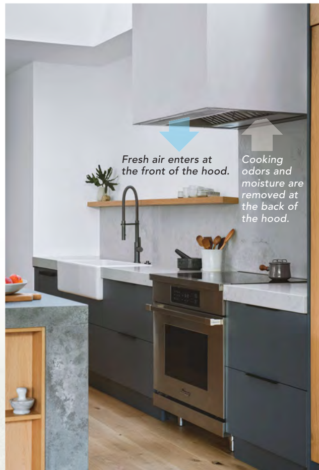
FRESH AIR FOR COOKING The kitchen makeup-air system replaces air exhausted by the range hood with filtered fresh air from outside. Also part of the air-quality strategy, the induction range avoids the many toxic byproducts of a gas combustion range.
