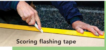
It's easier to work with sticky flashing tape when a portion of the release liner is left on. This keeps the tape from getting stuck to itself or to sur-
