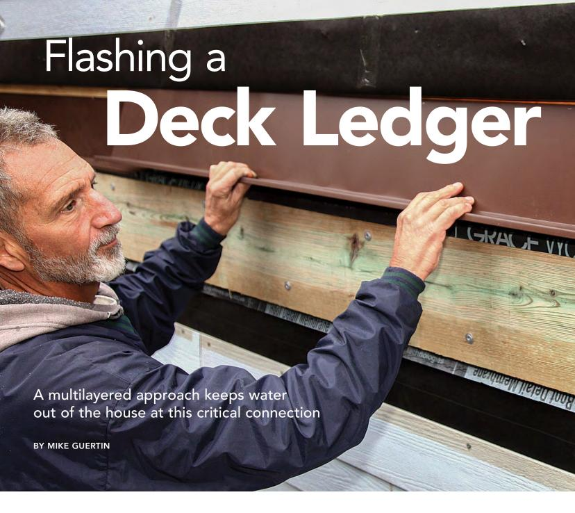
've dismantled many old decks in preparation for building new ones. In several cases water that leaked around insufficient ledger flashing or through holes in the flashing caused the rim joists to deteriorate. Fortunately the rot on those homes was limited and didn't lead to any deck collapses. But given more time, the water leaks and decay could have led to the ledgers loosening and not being able to support the deck.
