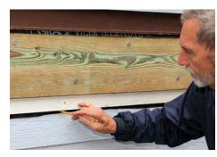
left 3 in. of space, just enough for the 1-in. decking and required 2-in. air space above the decking.
