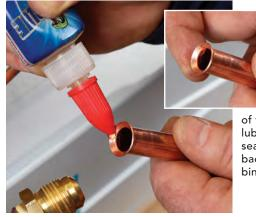
Apply a thin coat of refrigeration oil or assembly lubricant such as Nylog to the front and back
