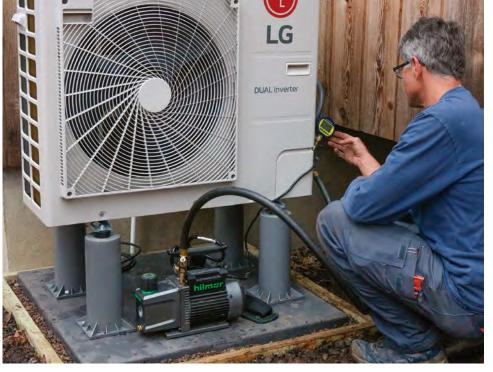
**3 THE VACUUM DECAY TEST** is done just before filling the line sets with refrigerant. At this point, the line sets have been pumped down into a deep vacuum to remove air and moisture. The vacuum level is measured with a sensitive micron gauge. To pass this test, the system must hold the deep vacuum after the pump is turned off.
