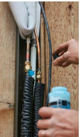
THE BUBBLE TEST is done while the system is under pressure, and is more sensitive to small leaks than the standing pressure test. For the bubble test, an approved leak-testing solution is sprayed or dabbed on the flares. If after about 10 minutes bubbles form, this means a leak is present and the flare must be re-done.
