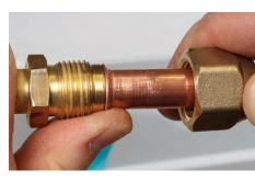
LINE UP THE FITTING Align the copper flare with the brass flare cone.
