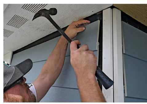
LOCK IN THE TOP Cut the top course to fit, and secure each piece with nails placed along the cut edge. The nail heads will hold the siding to the wall, and the shaft of the nails will keep it locked to the siding below it.
