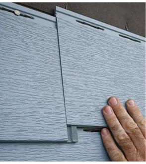
SLIDE IN THE JOINT Each piece connects to the piece to its left via a rabbeted half-lap joint. Tap the siding into place so that the bottom connects to the piece below.
