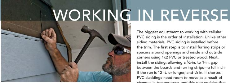
NAIL EACH COURSE Once a piece of siding is set in place, secure it with 1<sup>3</sup>/<sub>4</sub>-in. stainless-steel roofing nails driven into the center of the nail slot every 16 in. and left a little loose.
