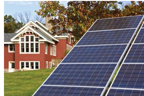
Lightening the load. The cost of operating the home’s geothermal system is offset by a 2kw photovoltaic array mounted beside the house.
