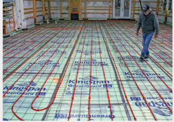
**Walk the area.** Just before the first concrete truck is scheduled to arrive, the entire floor area should be inspected to ensure that nothing will complicate the pour. This includes fixing loose radiant tubing, tenting mesh reinforcement, and any gaps that could allow concrete under the insulation, causing it to float.
