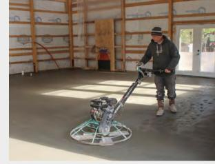
**FLOAT BLADES FIRST** Wide float blades or clip-on float pans spread the weight of the power trowel over a greater surface than trowel blades so the machine doesn't sink into the soft concrete. Once the bleed water has evaporated from a section, the operator floats the surface, which smooths it and brings up a layer of cement paste for later troweling.
