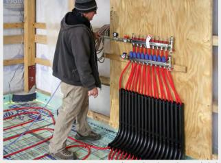
**Monitor pressure.** A test tee with a Schrader valve and dial air-pressure gauge is connected to the radiant manifold. As the concrete is placed, a stream of air from the tubing or a drop-in pressure at the gauge will indicate damage to the tubing that must be fixed before the pour can continue.
