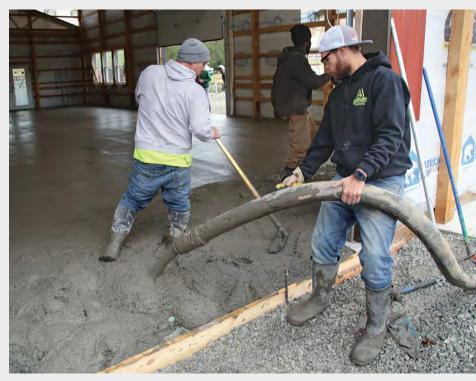
**WORK TOWARD THE EXIT** The crew continues placing, screeding, and bullfloating 16-ft. by 20-ft. sections, moving closer to the concrete pump. As less length is needed, the crew removes sections of the hose to make it lighter and more manageable.
