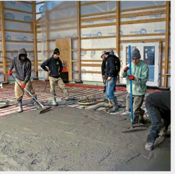
**LET IT FLOW** Once the concrete starts flowing, the pumping crew will try to maintain a 16-ft.-wide strip of concrete with uniform depth that matches the planned slab thickness. The pumping crew is helped by the finishing crew, which uses placement tools to spread the wet concrete to the right depth.
