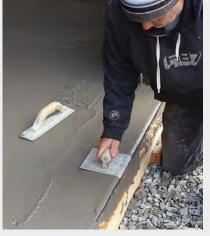
**EDGES COME FIRST** Bleed water often evaporates faster at openings because of sunshine. Once the surface has a matte finish, the crew will start finishing exposed edges, rounding the concrete corner by running the edger back and forth in 2-ft. to 3-ft. sections with the leading edge slightly raised.
