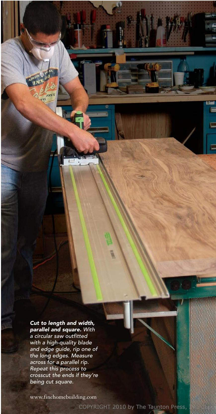
**Cut to length and width, parallel and square.** With a circular saw outfitted with a high-quality blade and edge guide, rip one of the long edges. Measure across for a parallel rip. Repeat this process to crosscut the ends if they're being cut square.
