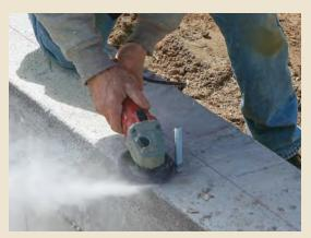
**GRIND SMALL LUMPS AND RIDGES** For bumps and lumps in the foundation surface, use a grinder with a diamond cup wheel to remove them.
