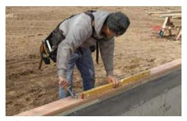
**TIGHTEN THE NUTS** Snug the nuts on the anchor bolts just enough to keep the mudsill layers level and flat. Use a 6-ft. level to check for flatness as you tighten, and do not overtighten the nuts, which can distort the sills downward and complicate subsequent framing.
