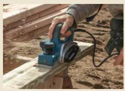
**SHAVE THE SILL** Plane the bottom of the mudsill to remove stock where the foundation is slightly high. A power planer makes the process fast and easy.
