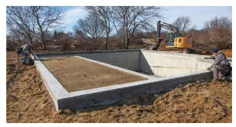
3:4:5 IS AN EASY CHECK To verify the walls are perpendicular to each other, use a 3:4:5 triangle to check a corner. From the corner point, mark a multiple of three along one wall and a multiple of four along the adjacent wall. The diagonal between the marks should be the same multiple of five.
