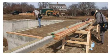
**SECOND SILL FOLLOWS SUIT** For the second mudsill layer we follow the same process as the first, with one crew member measuring the bolt locations and another drilling holes and cutting the sill pieces to length.
