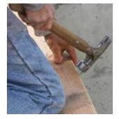
ALIGN AND NAIL After setting each piece on top of the treated layer, drive a few nails to help align and hold the lined-up layers together.
