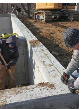
**MARK THE OTHER END** Pull a measurement from the first corner point and mark the length of the plate at the other end of the wall. Swing a line with a pencil against the tape. This provides a precise intersecting point for the perpendicular measurement. With the first wall laid out, measure over and mark the corners for the opposite wall, using the same setback for the stone veneer.
