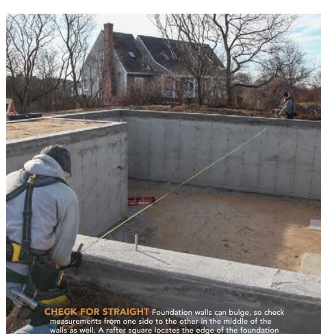
without the chamfer for an easier, more accurate measurement.
