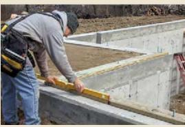
**FIT THE ADJUSTED BOARD** After planing the board, put it in place over the anchor bolts and then double-check the height adjustment with a level.
