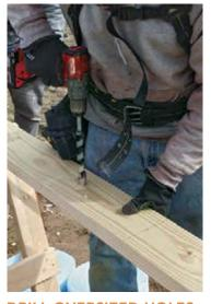
**DRILL OVERSIZED HOLES** Drill <sup>3</sup>/<sub>4</sub>-in. holes for <sup>5</sup>/<sub>8</sub>-in. bolts and <sup>5</sup>/<sub>8</sub>-in. holes for <sup>1</sup>/<sub>2</sub>-in. bolts. Keep the holes minimally oversized so you can use the bolts as a fulcrum to straighten warped mudsill stock.
