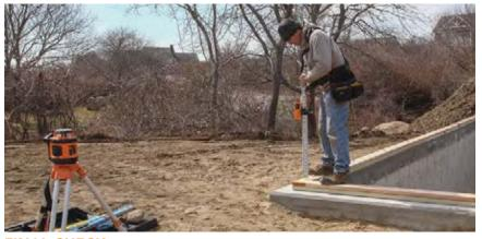
**FINAL CHECK** After the nuts are all snugged down, check the foundation for level once more with the laser. To make the process go more quickly, set the detector/receiver on the rod about <sup>1</sup>/<sub>8</sub> in. low. At each location, the <sup>1</sup>/<sub>8</sub>-in. gap between the rod and sill is easy to gauge.
