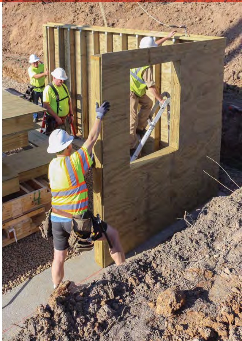
LIFT AND PLACE
