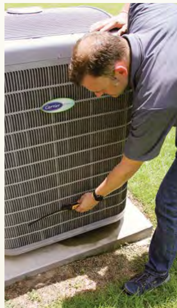
MEASURE REFRIGERANT TEMPERATURE I check the temperature of the refrigerant lines close to the outdoor unit with clamp-on thermometers from Fieldpiece. I sand the tubing first for an accurate measurement.
