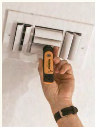
CHECK AIR TEMPERATURES Back inside, I measure the temperature of the air entering a large return-air grille as far away from the air handler as possible. Then I measure the air temperature from a supply grille as close to the air handler as possible. Finally, I measure the temperature of ambient outdoor air coming into the outdoor unit on the side opposite to the refrigeration lines.
