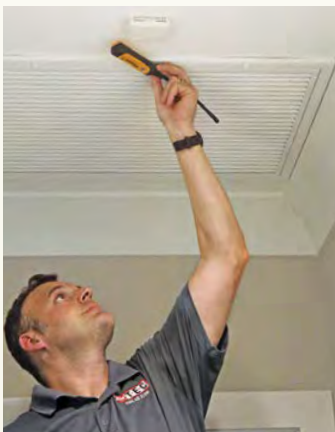
CHECK AIR TEMPERATURES Back inside, I measure the temperature of the air entering a large return-air grille as far away from the air handler as possible. Then I measure the air temperature from a supply grille as close to the air handler as possible. Finally, I measure the temperature of ambient outdoor air coming into the outdoor unit on the side opposite to the refrigeration lines.
