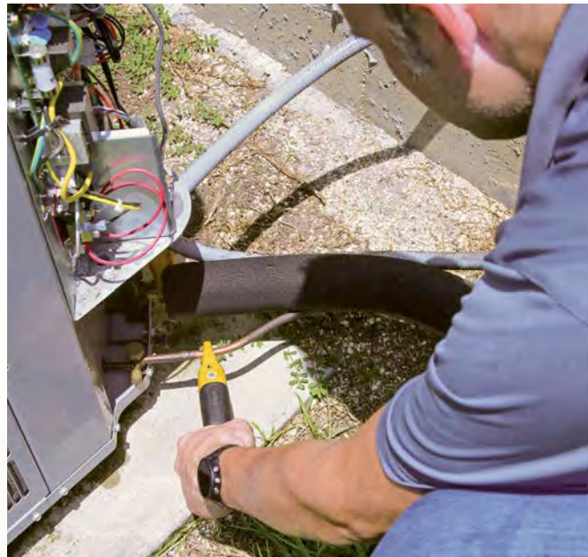
MEASURE REFRIGERANT TEMPERATURE I check the temperature of the refrigerant lines close to the outdoor unit with clamp-on thermometers from Fieldpiece. I sand the tubing first for an accurate measurement.
