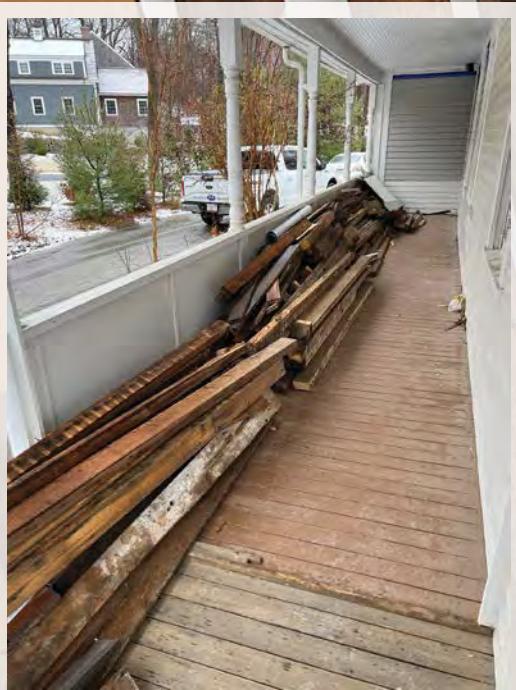
OUT OF THE WEATHER Plan ahead for a safe, dry place to bring the salvaged lumber as it is removed. A covered porch works well.
