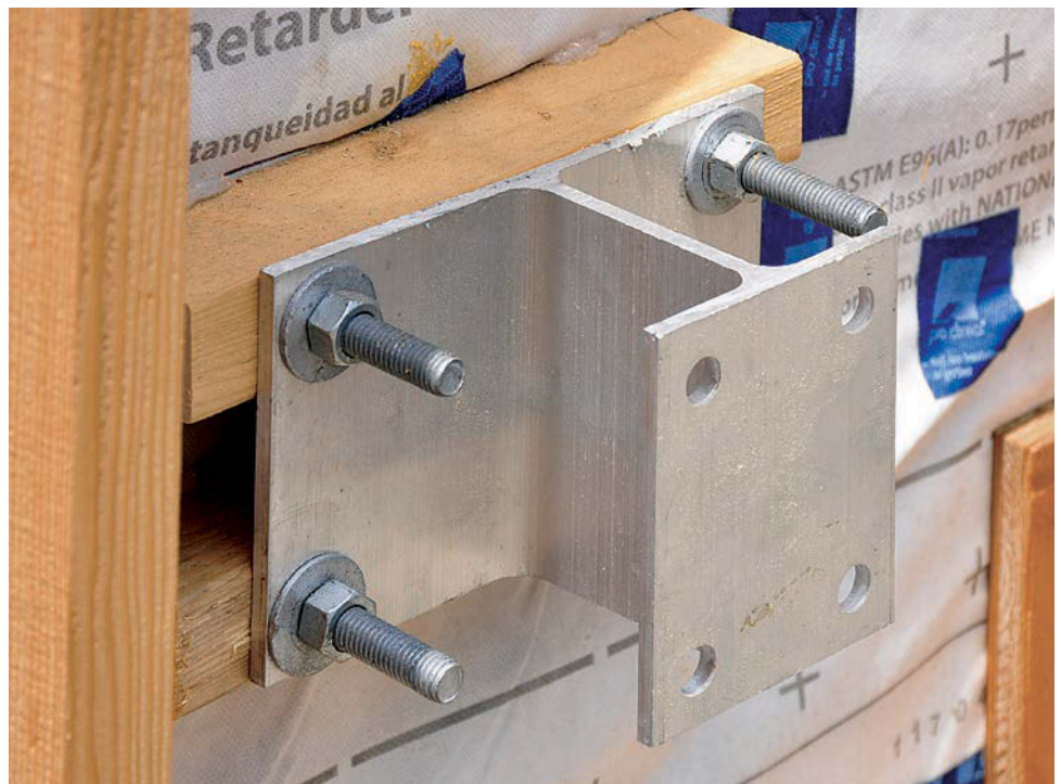
LEDGER-READY Ledgers can sometimes be attached directly to Larsen trusses. Another option is to use hardware like the Maine Deck Bracket spaced appropriately off the sheathing for deck and porch floor and roof attachments.
