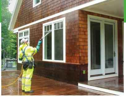
**APPLY BOTTOM TO TOP** Apply the brightener from bottom to top and allow it to work for a few minutes. Keep the surface wet to prevent the brightener solution from drying on windows, siding, or trim, which can leave persistent water spots.
