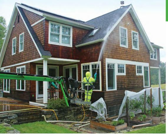
**WORK FROM THE BOTTOM UP** Chemical application and washing should start at the bottom of the building and move toward the top, because drips of old finish and stripper should fall on siding already wetted with the stripper solution.
