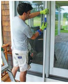
**REMOVE AND LABEL SCREENS** If you leave screens in place, you run the risk of residue from the old finish or water spots from cleaning chemicals on the glass. Label the screens and keep track of any hardware so the screens are easy to reinstall.
