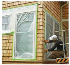
**COVER WINDOWS** Plastic masking film is cut to fit over windows for protection from stain overspray. The plastic is held in place with high-quality painters tape that won't leave a tape or adhesive residue even in damp or hot conditions.
