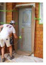
**PULL THE PLASTIC** Once a section is stained and has dried for an hour or two, remove the plastic sheeting and masking tape. When practical, do this work while bucket lifts or ladders are in position for staining to save setup time.
