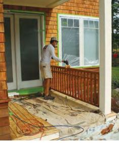
**PLAN WORK FOR BAD WEATHER** Covered decks and porches can be worked on in the rain and during dewy mornings. We use a finish that works with a moisture content up to 20%.
