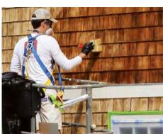
**WORK IN THE FINISH** Once the finish is sprayed on the surface, we brush it into the siding with a 5-in. Olympian block stainer brush. This ensures the oil is fully worked into the wood and moves excess stain from less to more absorbent wood grain.
