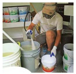
**MIX THE STRIPPER** The stripper must remove any surface contaminants and all the old finish without damaging the underlying wood. We mix it in batches, adjusting the concentration to match the existing finish. We start with about 1 cup of stripper to 1 gal. of water.
