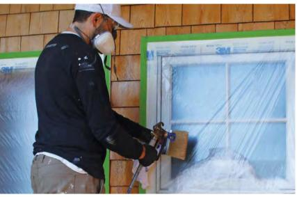
**SPRAY**—**DON'T DIP** We load the brush with stain using a quick, gentle spray from the spray nozzle. This method is faster, less messy, and more convenient than managing a paint pail or can of stain to wet the brush.
