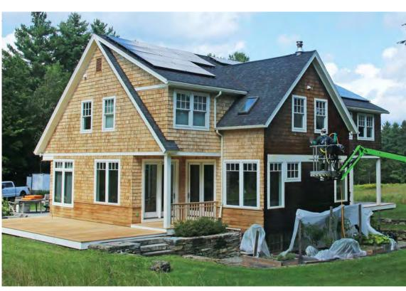
**READY FOR FINISH** Stripping and brightening continues by elevation. Once all sides of the house are stripped and brightened, the siding is allowed to dry for two or three days without rain before finishing. Ideally, the siding should be at about 15% moisture content before staining.
