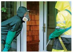
**TEST EFFECTIVENESS** We test the stripper on a small section under a porch or overhang where the siding hasn't been washed by rain. We repeat this test on every elevation, as each will have different amounts of dirt and old finish. A ratio of 1<sup>1</sup>/<sub>4</sub> cup stripper to 1 gal. of water was effective on most of this house.
