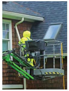
TAKE DOWN DOWNSPOUTS Downspouts prevent the cleaning solutions and finish from reaching the siding reliably, so they have to come off. We replace downspouts after every work day so the house's water-management system is fully intact for storms.
