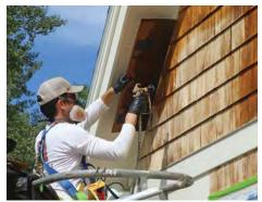
**PROTECT PAINTED SURFACES** A cardboard spray shield prevents stain from getting on trim and other painted parts of the house. The cardboard becomes quickly saturated with stain, so we use multiple shields and allow them to dry before re-use.
