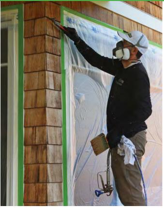
**KEEP A WATCHFUL EYE** As you work on a section, look for drips of stain and wipe them away. Also look for drips from previous coats of finish and scrape these off as you go. Removing them later will damage the new finish and may necessitate recoating.
