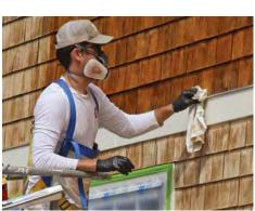
WIPE DRIPS AND OVERSPRAY Painted trim like this frieze board doesn't need to be masked, but the oil finish must be wiped off before the stain dries. If the finish is partially dry and resistant to wiping, it can often be cleaned off with mineral spirits.
