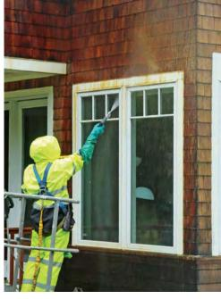
**SPRAY ON THE STRIPPER** A pump permanently mounted in the trailer transfers the concentrated stripper to the spray nozzle. We thoroughly wet the siding surface with the stripper and then allow it to sit for a few minutes, described as dwell time.
