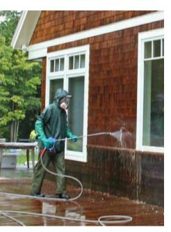
**RINSE THE BRIGHTENER** After about 5 to 10 minutes, we rinse off the brightener with another soft wash of water. Work from the top down to prevent streaks and water spotting. Keep windows wet to avoid those water spots.
