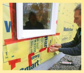
WRAP IT UP Cut a 6-in. to 12-in. strip of housewrap about 6 in. longer than the window width. Apply a piece of housewrap tape or flashing tape along one edge with no more than 1 in. of adhesive above the edge of the housewrap strip. Tape the strip to the bottom flange, making sure the adhesive of the tape doesn't seal onto the flashing pan that's behind and below the window flange.
