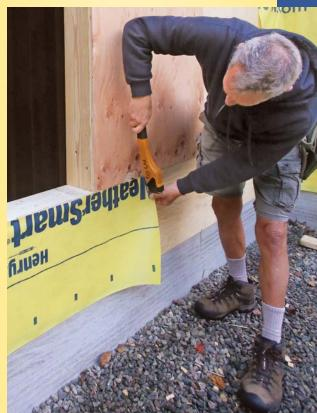
STAPLE UP THE APRON Cut a piece of housewrap 2 ft. longer than the rough opening is wide. Position the sheet flush with the rough sill and centered so that 1 ft. extends past either side of the rough opening. Fasten along the top edge. Leave the bottom of the sheet loose if an inspection is required or roll the sheet up and tack-fasten at the ends.
