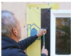
**SEAL THE SIDES FIRST** Seal the flanges to the housewrap jamb strips at the sides first, and then the head, with flashing tape. Leave the bottom flange open to allow water collected by the sill pan to weep and dry.
