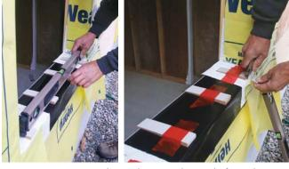
**LEVEL THE SILL** Use shims (these can be made from the same material you used to slope the sill) to create a flat surface for the window to sit on. Move the shims in and out until they are level and aligned to establish a base for the window, then tape them in place. Now is a good time to dryfit the window and check to make sure you can get it level and plumb in the opening.
