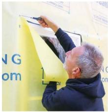
ROLL OVER THE WINDOWS Install the housewrap as usual and when you get to a window, just keep going. Fasten the housewrap along the top edge, letting it drape over the window, but don't fasten too close to the window just yet. Cut out around the windows with scissors or housewrap slitters, or carefully with a knife. Then fasten the housewrap to the walls, and seal the edges.
