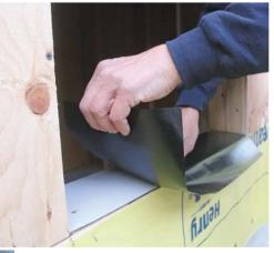
**SEAL THE SLOPE** If you are going to slope the sill, you need to remember to drop the rough sill the thickness of the material you are using to create the slope. Once installed, the beveled siding is covered with flashing tape (or fluidapplied flashing) that laps onto the apron.
