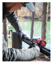
Trouble-free tensioning. The cables in each rail section can be tightened simultaneously using the two impact-driver-operated tensioners located inside the top rail.
