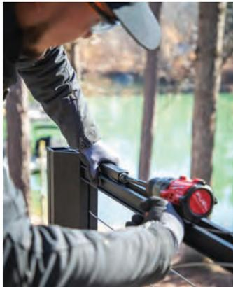
**Trouble-free tensioning.** The cables in each rail section can be tightened simultaneously using the two impact-driver-operated tensioners located inside the top rail.
