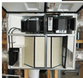
V IS FOR VENTILATION Many HVAC experts agree that it is best to separate ventilation from heating and cooling ductwork. Like the installation shown here, independent ductwork allows the ERV to perform as designed and commissioned.
