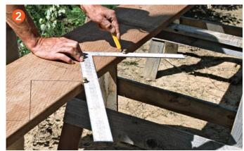
Stair buttons ensure an accurate layout. Small clamps known as stair buttons screw onto a framing square to mark the unit rise and the unit run on a stringer. Working from bottom to top, slide the square up the stringer, marking each notch the same way.
