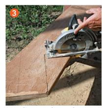
Start the cuts with a circular saw. Cut the notches on the waste side of the line. Stop the blade just shy of the intersecting line, and finish the cut square and plumb with a jigsaw, a handsaw, or a reciprocating saw.
