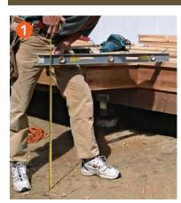
**Determine total rise.** Use a level and a measuring tape to find the total rise. Remember to factor in a concrete pad if one will be installed later. Use the calculations explained above to figure out the number of steps and the total run.
