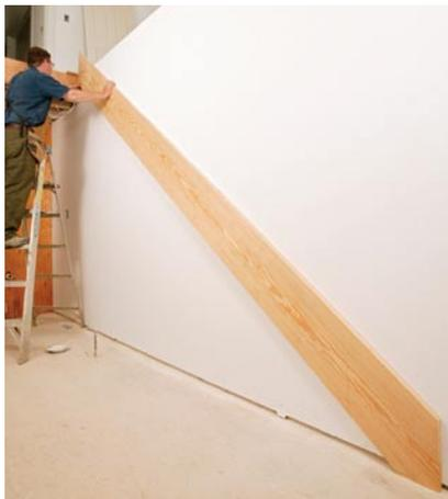
**Test-drive before the cut.** Before routing the stringers, check the fit of the stringer at the upper and lower landings. A wood scrap the same thickness as the flooring helps to determine the fit.
