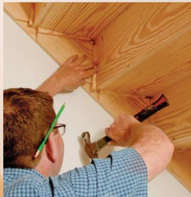
Treads and risers that are glued and wedged into routed stringers are tighter and more stable than conventionally framed stairs
