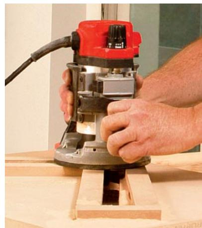
**Use pieces of scrap to create a routing template.** After drilling a pilot hole, use a top-bearing straight bit with the same ½-in. radius as the tread's nosing to rout out the template. Pop the ½-in. material and nails off the jig, and you're ready to go.
