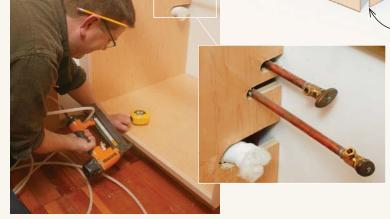
**A great reason for backless cabinets.** A backless cabinet can be placed and easily scribed to any protruding plumbing or wiring. The base cabinets are sized to create a traditional 3-in.-deep kick space below. Once the cabinets are attached to the base, the face frames are applied.
