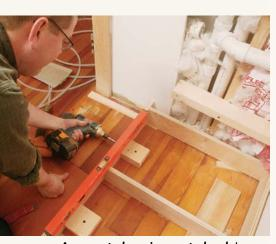
A separate base is easy to level. In older houses, it's often easier to build and install separate bases for the lower cabinets. Basically plywood boxes, the bases are shimmed level and attached to the floor. Plywood strips attached to the top of the cabinets support the countertop.
