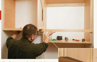
**Check your work.** A handy layout and construction tool to use on jobs like this project, a story stick is a length of plywood scrap on which room measurements are recorded and cabinet spacing is determined. Once the cabinets are installed, use the stick to doublecheck their locations.
