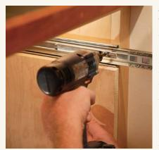
Systematic approach to drawer slides. Allow 1/4-in. clearance between drawer fronts. Mark drawer-bottom locations on the inside cabinet wall, then transfer these marks to a piece of plywood. Use this piece inside the cabinet to support the top drawer slides while they're being attached to the cabinet sides. In turn, cut it down to the next drawer-slide height for each drawer. For the bottom drawer, rest the slide on a scrap of 1/4-in. plywood on the bottom of the cabinet.
