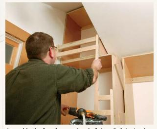
**Assemble the face frames ahead of time.** Built in the shop with pocket screws, the frames are scribed to the wall and nailed to the boxes as units.
