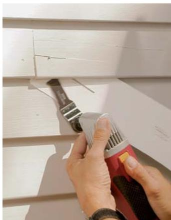
**Cut stubborn nails.** Use a multitool outfitted with a metal-cutting blade to cut nails that won't pop. To protect the clapboard and the housewrap beneath, insert a piece of coil flashing stock between the boards, then brace the tool on the wall and carefully cut the nail. Stubborn nails with small heads also may be driven through the board with a nail set.
