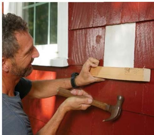
**Hide the new nails.** After cutting a replacement shingle, insert the new piece in place until it's ¼ in. below the course line. (The top may be trimmed a couple of inches to accommodate nails in the course above.) Drive two stainless-steel ring-shank nails just below the course line above. Then use a nail set to drive the heads flush. With a block, drive the shingle up until it's even with the course line, which also pushes the nails up under the course above.
