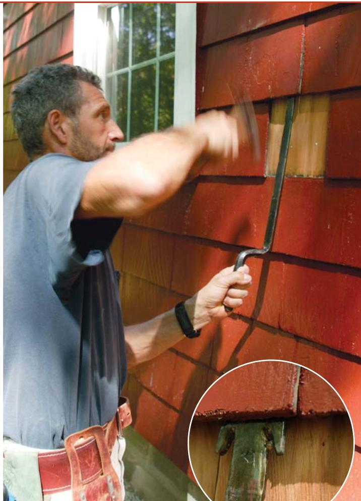
**Clear the nails.** A slate ripper is a great tool for pulling concealed nails. Slide the flat blade beneath the overlapping shingle, tap it sideways so that one hook grabs a fastener, and then tap downward on the strike arm of the ripper's handle. The hook either pulls out the fastener (inset) or cuts through it.
