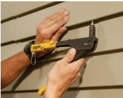
Vinyl also can be patched temporarily with an overlay that covers the damage. From a long-enough piece, cut the hem off the top and the upturned edge of the butt lock. The patch slips beneath the butt-lock joint above, and the bottom overlaps the joint below. Drill and snap two pop rivets into the butt lock at the bottom to hold the piece in place.
