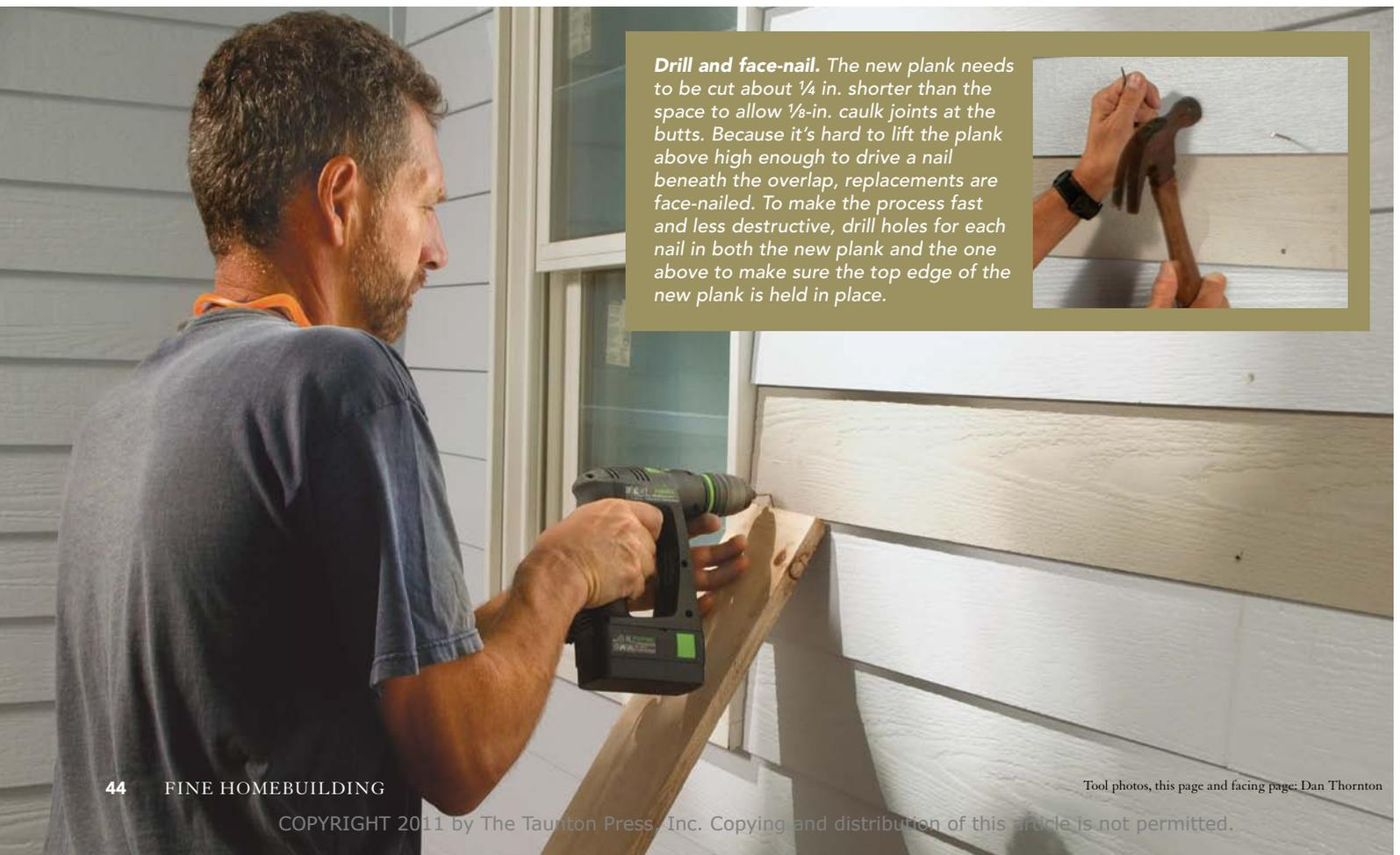
**Drill and face-nail.** The new plank needs to be cut about  $\frac{1}{4}$  in. shorter than the space to allow  $\frac{1}{8}$ -in. caulk joints at the butts. Because it's hard to lift the plank above high enough to drive a nail beneath the overlap, replacements are face-nailed. To make the process fast and less destructive, drill holes for each nail in both the new plank and the one above to make sure the top edge of the new plank is held in place.
