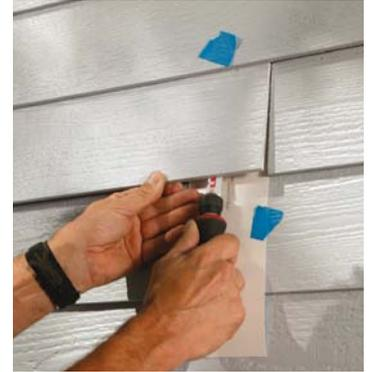
Slide a thin flat bar under the fiber-cement plank, and pry it up about  $\frac{1}{8}$  in. so that the cutter can reach the shanks. A hidden-nail cutter (left) has fairly thin, deep jaws that slip between planks. Alternatively, nails can be cut with a metal-cutting blade mounted in a recip-
