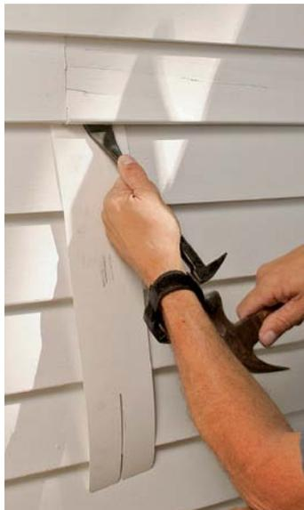
**Pop the nails.** Use a thin-bladed flat bar to pry up both the damaged clapboard and the clapboard above it, about 1/4 in. at each nail position. A piece of aluminum or plastic flashing stock protects the clapboard below from being damaged during the process. Usually, when the board is tapped back down, the nail head remains proud, ready to be pulled. If it's apparent that a nail isn't moving, stop prying.
